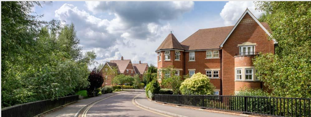
Southern entrance into Frenchay Road looking north west from the southern canal bridge
